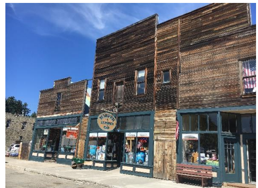
Wood-frame commercial structures
